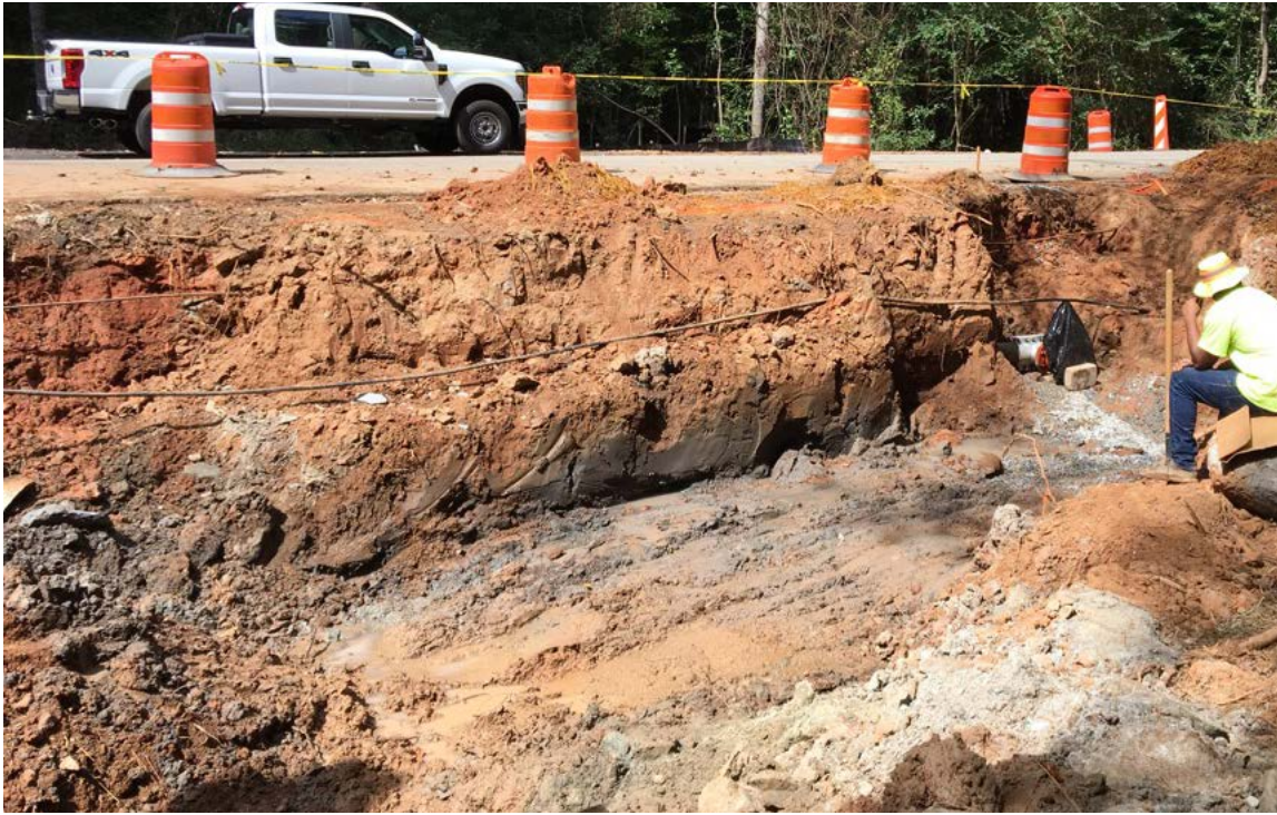
Photo 1: Excavation began for the 8" waterline installation.
