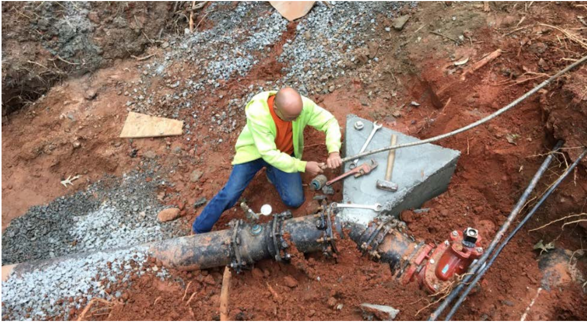
Photo 1: The new waterline is undergoing pressure testing.
