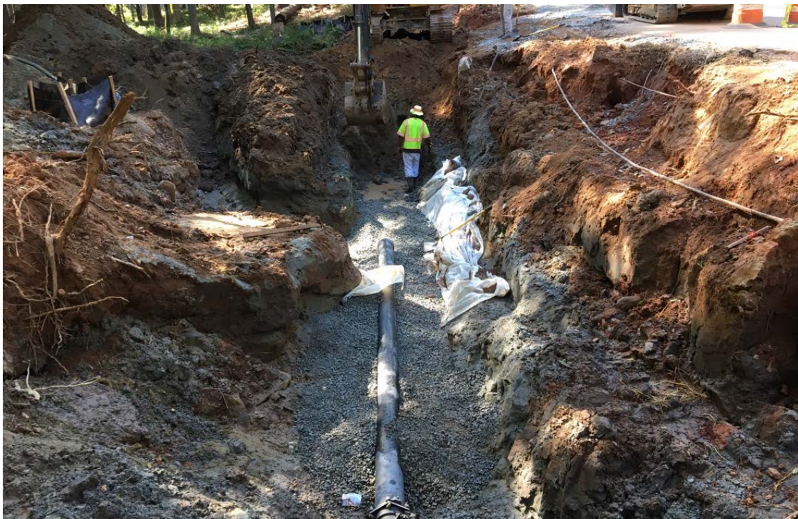
Photo 2: Excavation resumes again allowing for installation of remaining new pipe.
