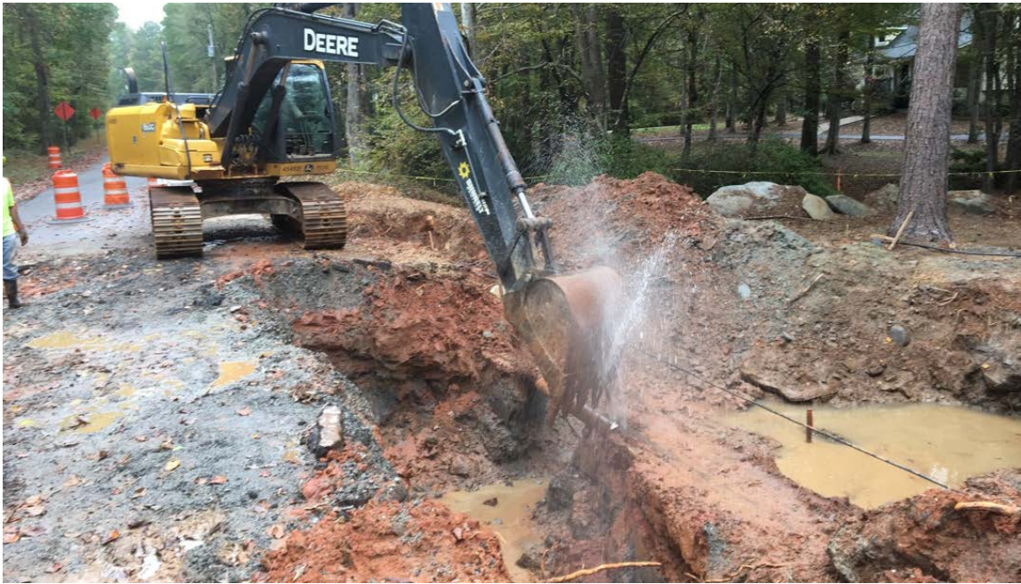
Photo 1: The waterline is removed.
