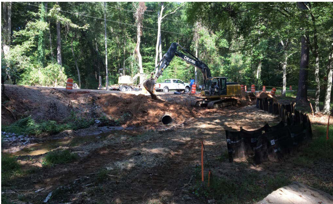
Photo 2: Excavation began today for the waterline relocation.
