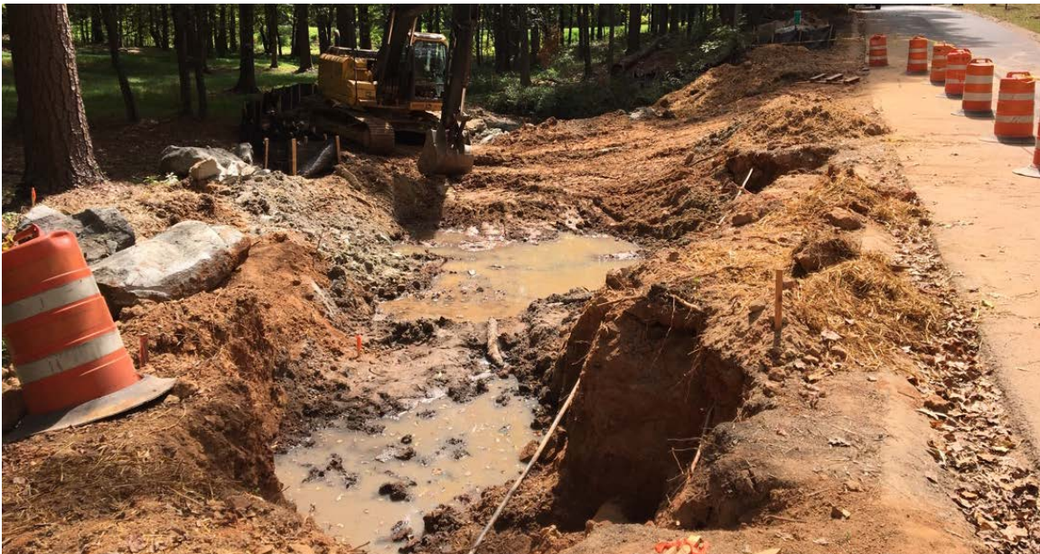
Photo 2: Excavation continues within the waterline pipe installation area.
