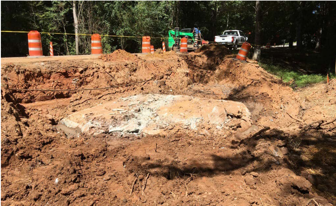
Photo 1: Today, work begins on breaking up the rock.
