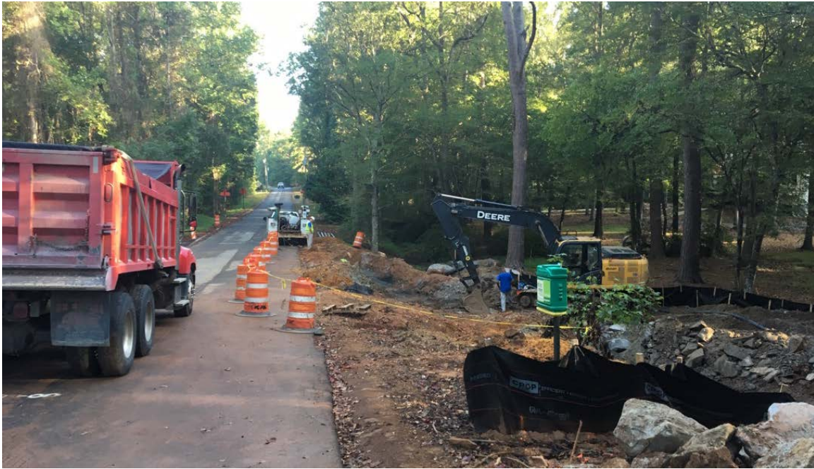
Photo 1: Overall work site.
