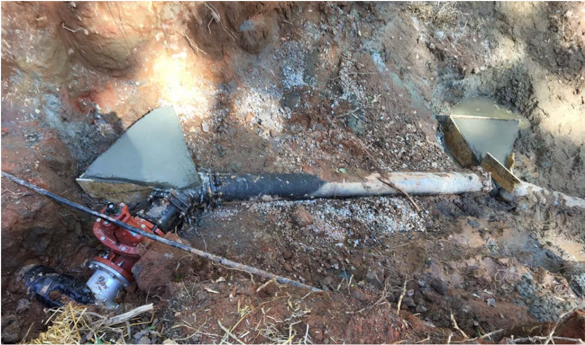
Photo 1: Thrust block constructed at 45 degree fittings.
