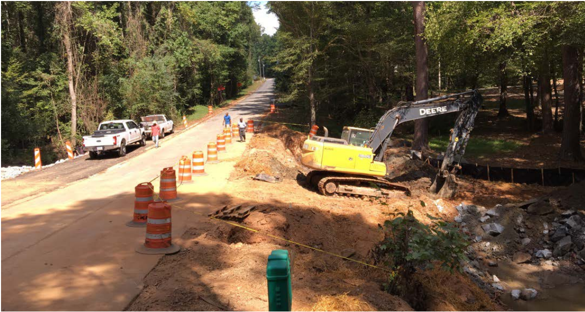
Photo 1: Rock debris is being removed from the construction area.
