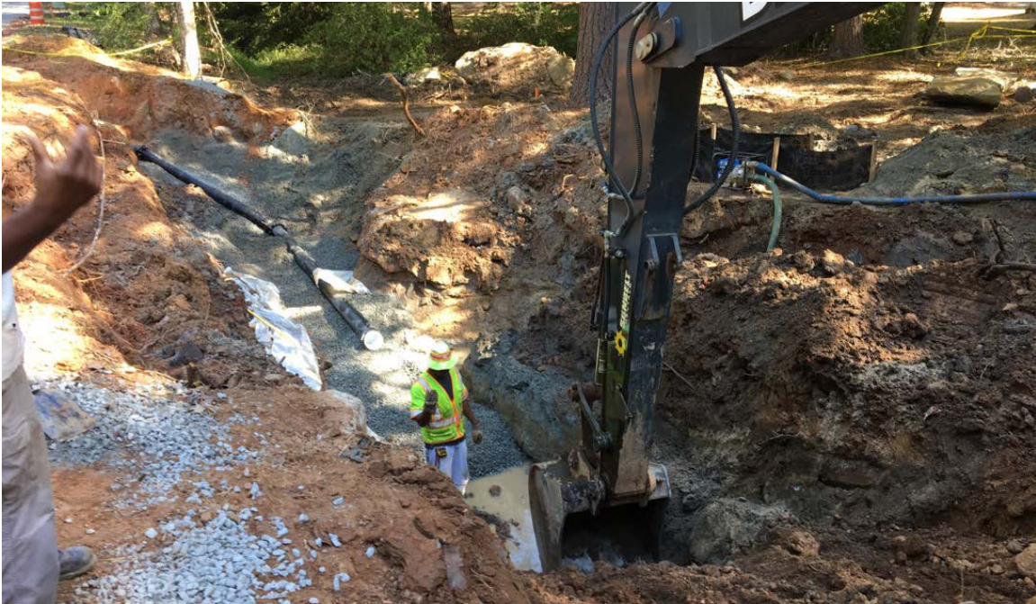
Photo 1: Excavation resumes again allowing for installation of remaining new pipe.
