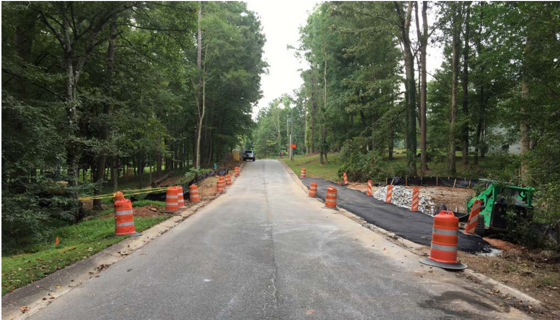
Photo 1: Construction of the temporary detour road is complete.
