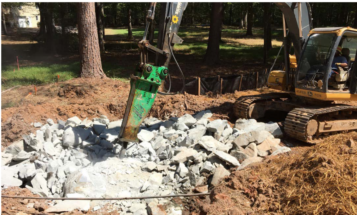
Photo 2: Progress is visible as demo continues on the large rock.
