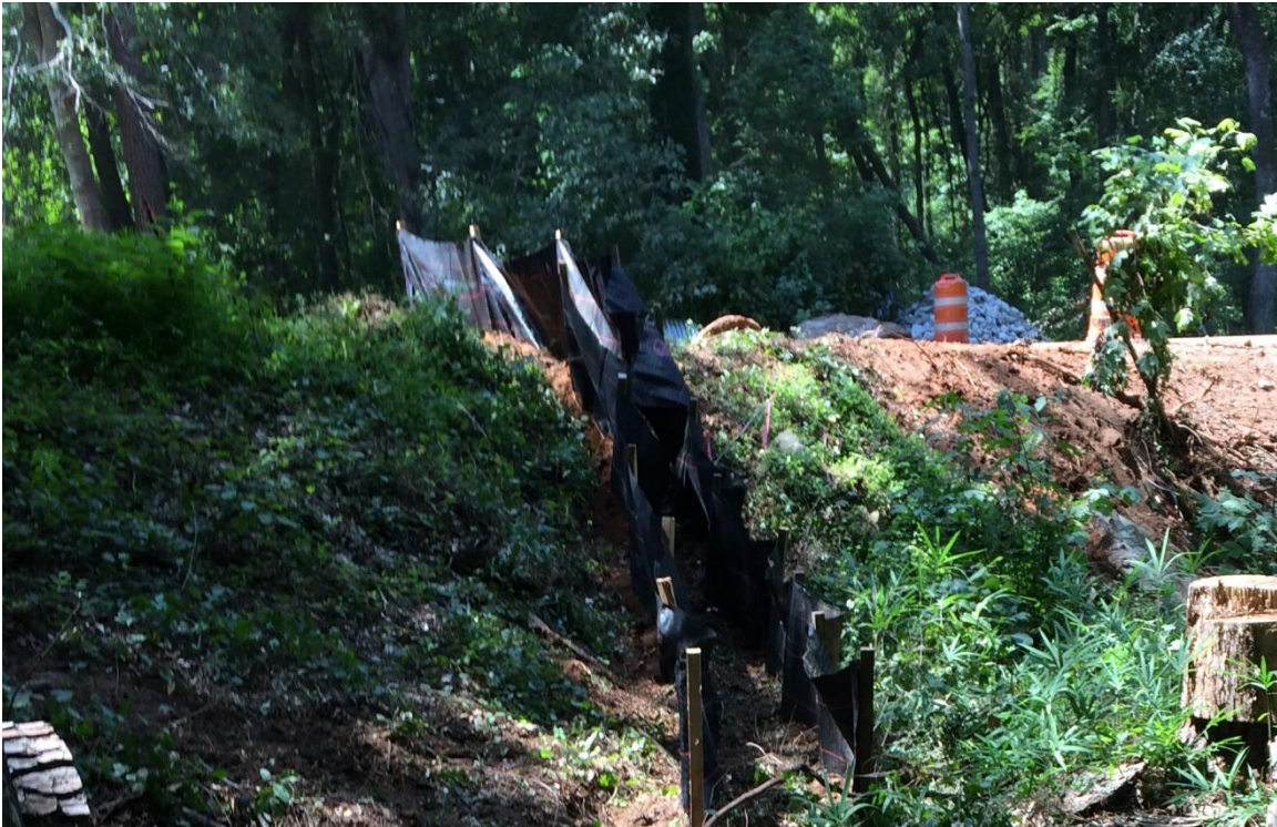
Photo 1: The last silt fence was installed. (August 15, 2018)
