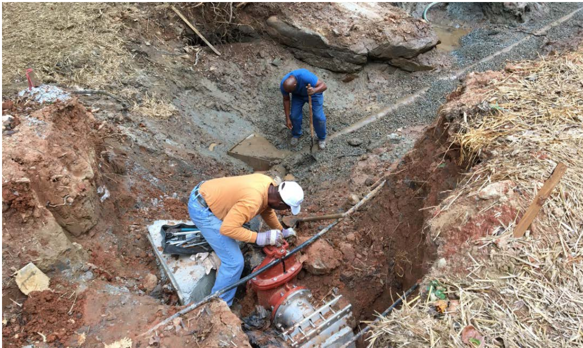
Photo 2: Work crews are tightening fittings where a leak is suspected.
