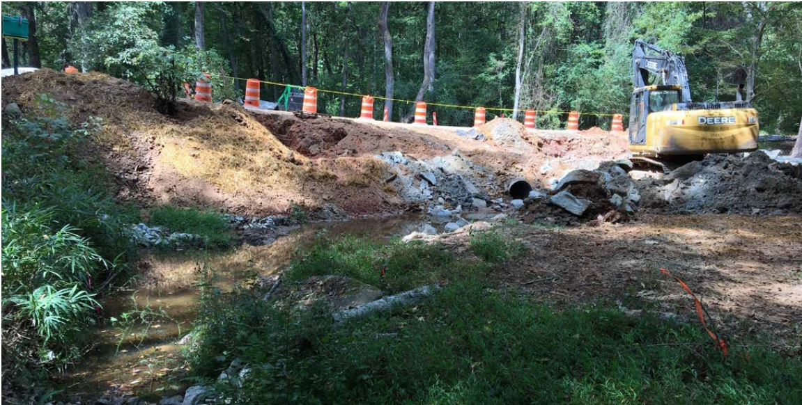
Photo 1: Work site overview.
