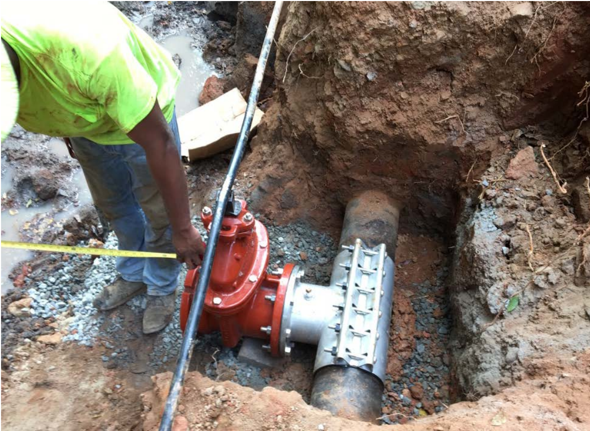
Photo 1: Installation of 8" x 8" tapping sleeve with valve has been completed.
