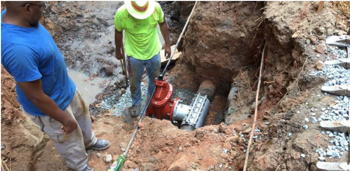
Photo 2: The wet tap is scheduled for the following day.
