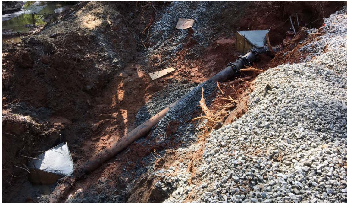
Photo 2: The thrust blocks were placed using a high-strength concrete mix.
