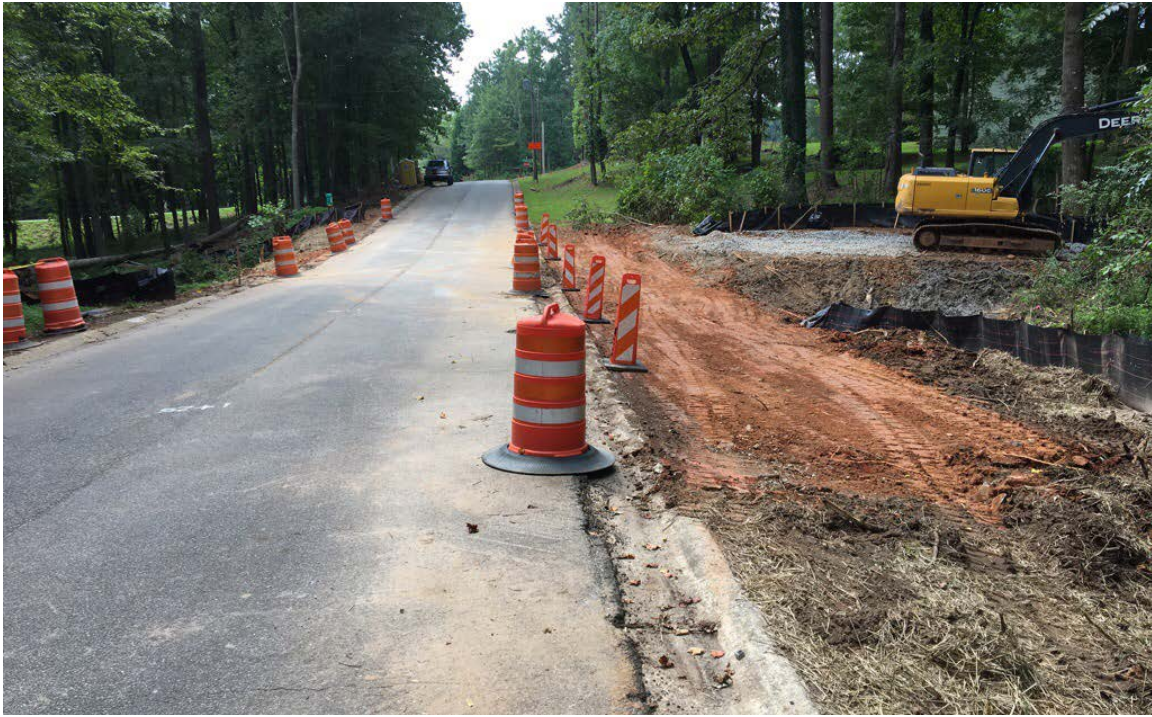
Photo 1: Construction of the temporary detour road is in progress. (August 24, 2018)
