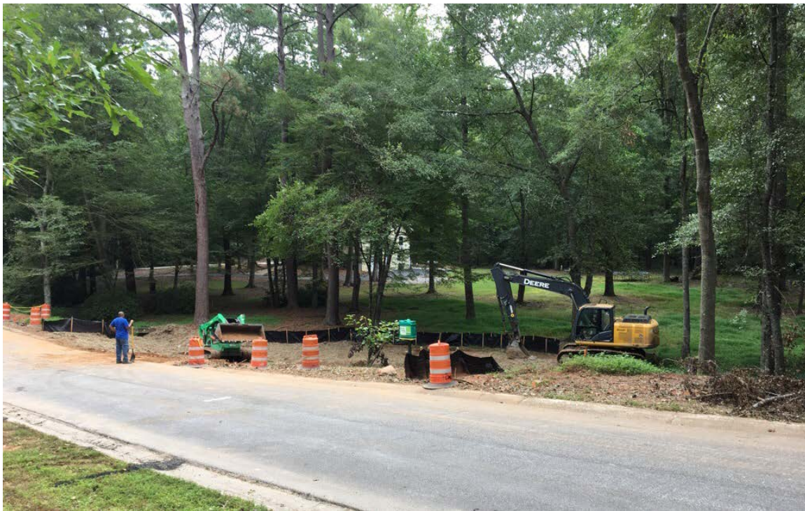
Photo 2: Disturbed areas near the existing culvert outlet have been stabilized with grass seed and hay.
