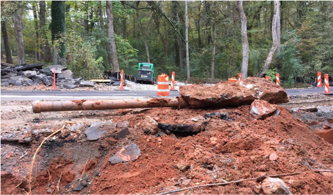
Photo 1: The portion of the existing (old) waterline has been removed.
