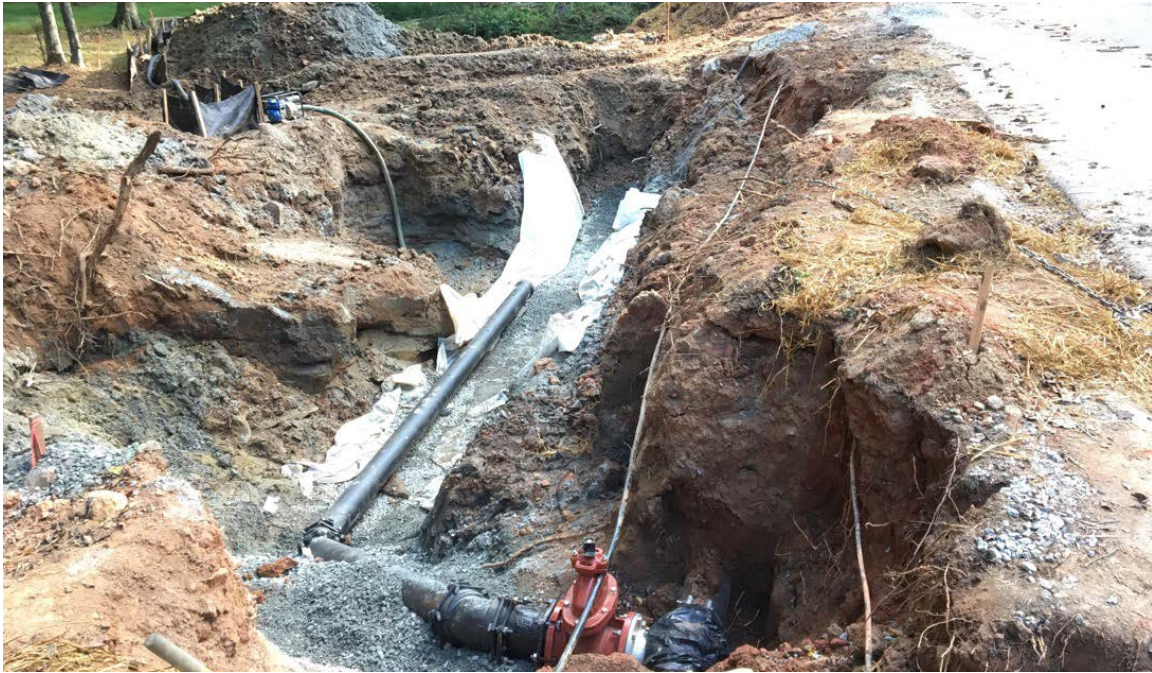
Photo 1: Approximately 36 feet of the new 8" waterline pipe has been installed.
