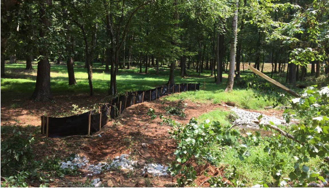
Photo 1: Silt fence is being installed around the construction site. (Monday, August 13, 2018)
