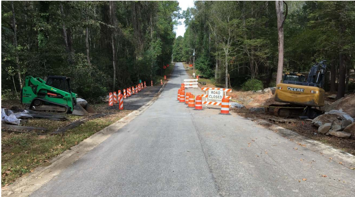
Photo 2: Overall site conditions.
