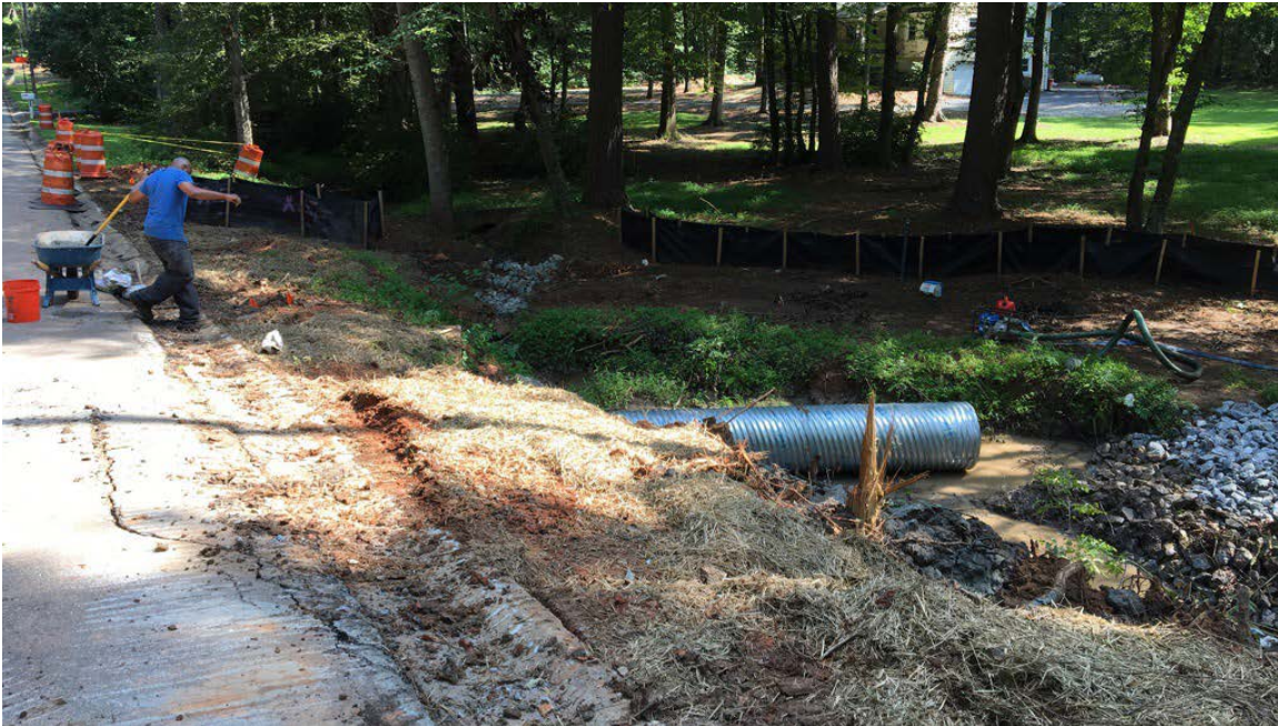
Photo 1: Diversion pipe installation.
