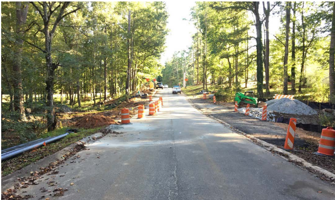
Photo 2: Overall work site.
