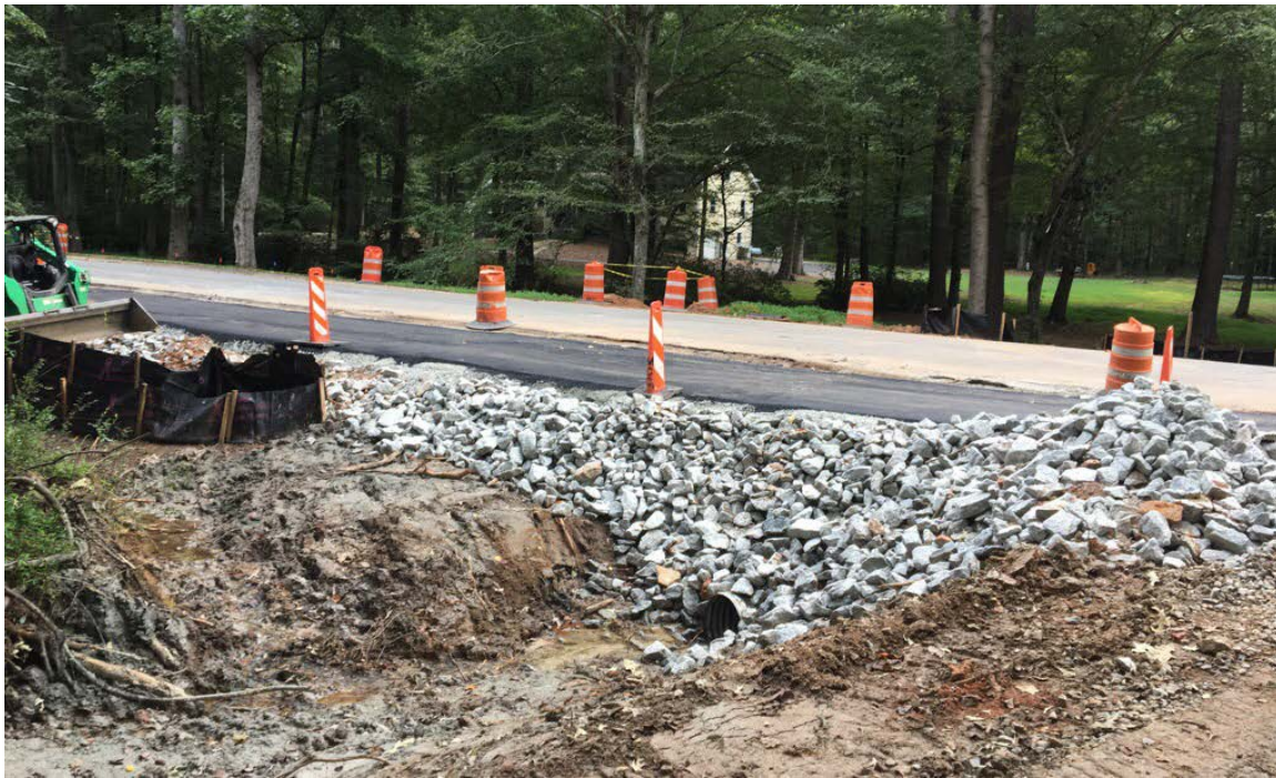
Photo 2: Construction of the temporary detour road is complete.
