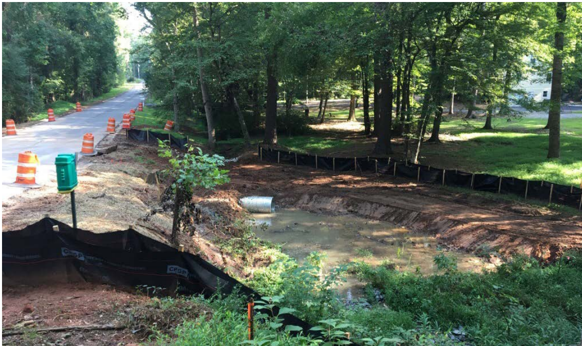
Photo 2: The temporary diversion pipe construction is complete. (August 23, 2018)
