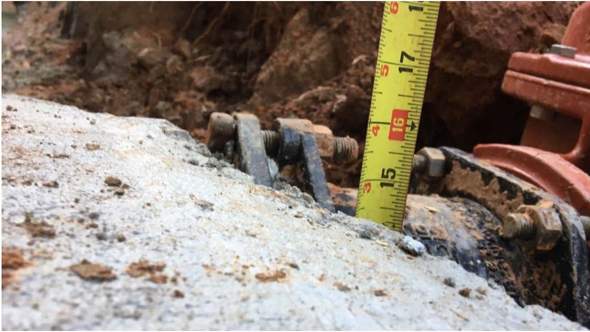
Photo 1: The thrust blocks are measured to verify they meet the County's specs.
