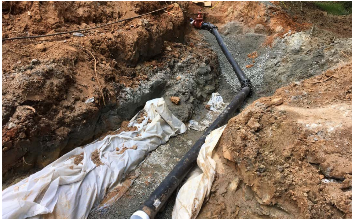
Photo 2: Approximately 36 feet of the new 8" waterline pipe has been installed.
