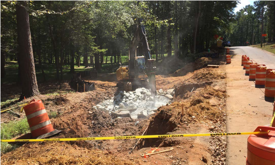
Photo 1: Progress is visible as demo continues on the large rock.
