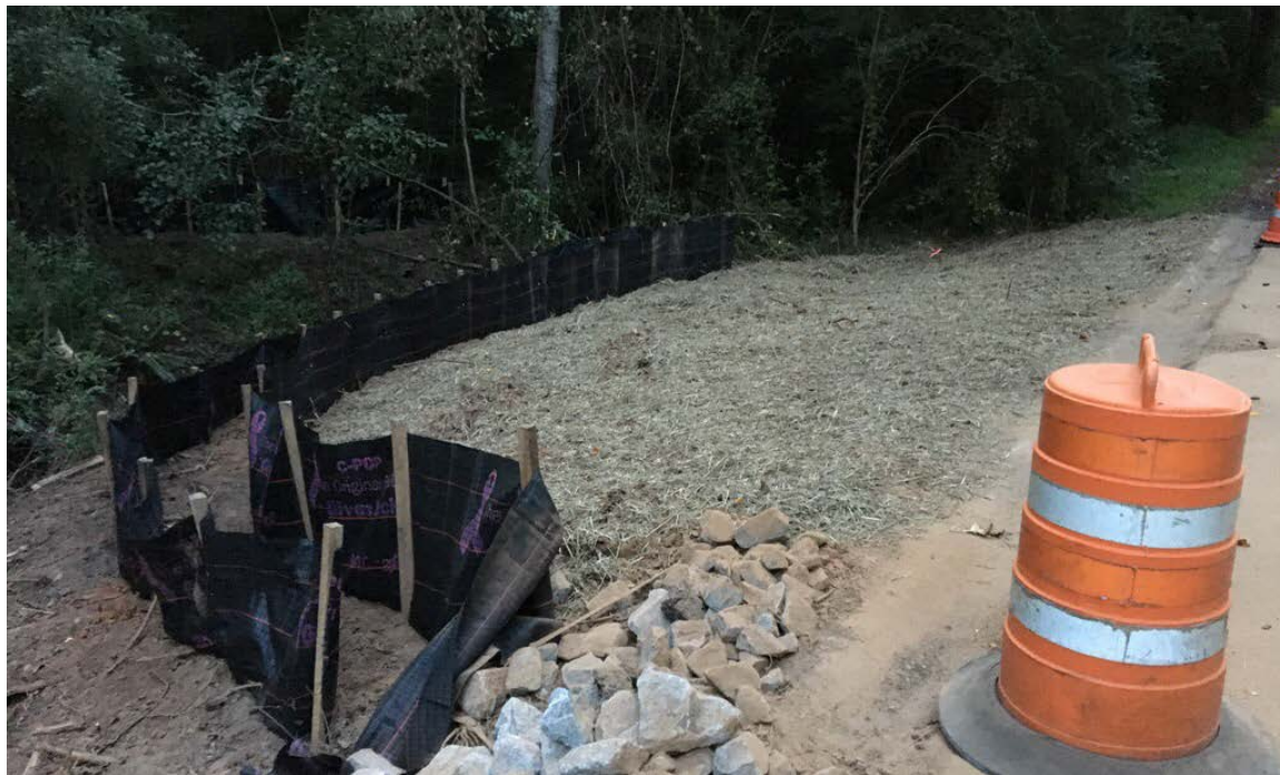
Photo 2: The disturbed areas on the west shoulder of Broom Boulevard are covered with mulch/hay/grass.
